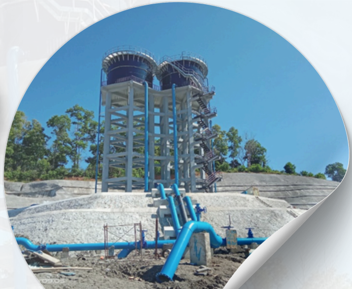
Installation Header inlet/outlet Pipe to Water Tower PT. MOS Purwakarta
