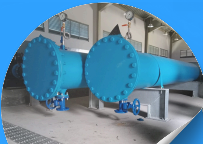
Installation Header Pipa GIP Diameter 600mm, Discharge Pump, PT. MOS Purwakarta
