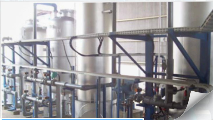
Demineralizer Plant, Capacity : 25 m 3 /h
