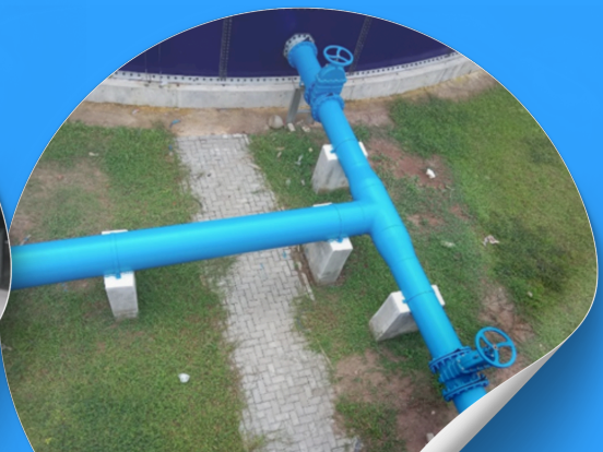
Installation Header Pipa GIP Diameter 600mm, Discharge Pump, PT. MOS Purwakarta
